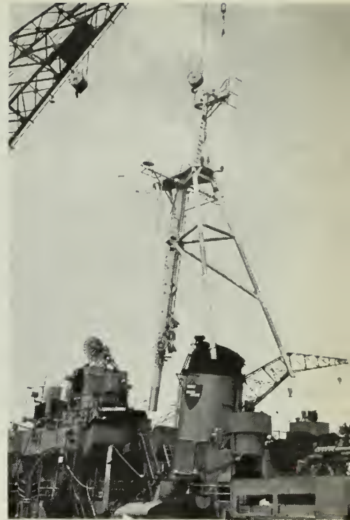
SHIP'S MAST—Crane at Pearl Harbor Naval Shipyard moves new mast into position on USS Cogswell (DD 651).
